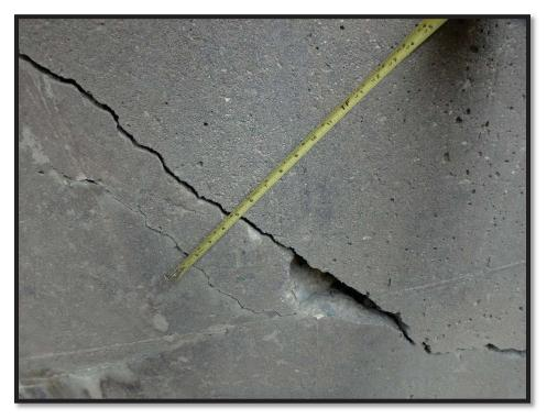
Photo 7 NE Wingwall, showing 3/8 to 1/2-inch crack with spalling in between migrating smaller crack, refer to photo 6
