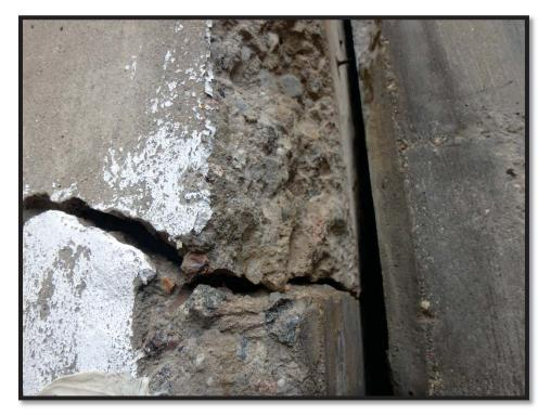
Photo 8 NE Wingwall, showing 1/2-inch crack at culvert joint, crack appears to be deep. Also showing spalling/scaling, refer to photo 6
