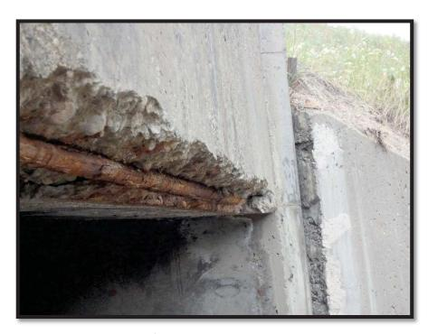
Photo 26 Bottom edge of top slab at south send, major spalling with exposed rebar along entire edge
