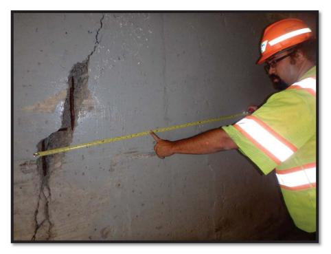
Photo 22 West Wall at 22-ft from south, showing diagonal shear crack ranging from 1/8 to 4-inches, migrating from top to bottom, spalling
