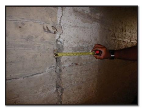
Photo 21 West Wall at 48-ft from south, showing multiple migrating cracks varying between 1/8 to 2-inches
