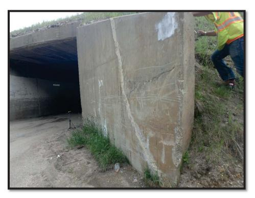
Photo 2 NW Wingwall, showing 1 large diagonal sealed fracture extending from top to bottom of wing and 1 smaller sealed horizontal crack
