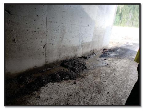
Photo 24 East Wall at south end showing concrete deterioration and section loss at bottom for several feet, heaving leakage
