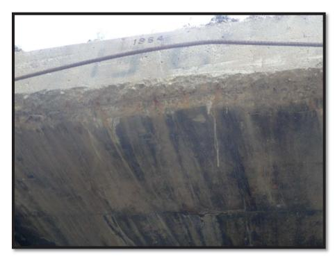
Photo 9 North headwall/edge of top slab, exposed rebar, concrete at bottom spalled off at edge. Also showing scrapes from live load.
