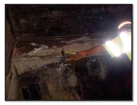
Photo 17 Top Slab at 90-ft from North (EB median), showing efflorescence, delamination, unsound and spalling, and large crack migration throughout entire top slab down through wall
