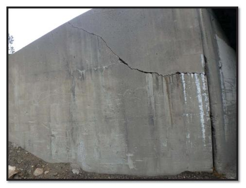
Photo 6 NE Wingwall, 1 diagonal crack extending from top to culvert joint, other vertical and horizontal sealed cracks migration
