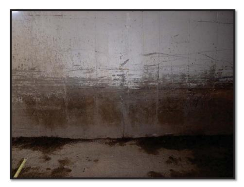
Photo 11 West wall, vertical 1/4-inch shear crack migrating from top to bottom located at 26-ft from north end
