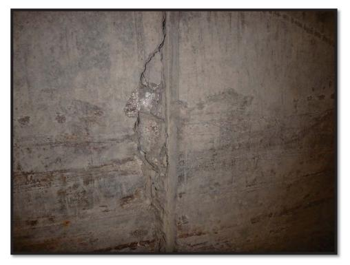
Photo 14 East Wall at 44- from North, spalled concrete. Construction joint not shown at this location on plans
