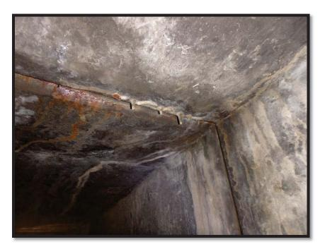
Photo 15 East Wall/Top Slab at construction joint 53-ft from North. Actively leaking and showing stalactites, efflorescence, delamination
