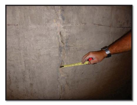
Photo 19 West Wall at 50-ft from south, showing vertical 1/2 to 3/4-inch shear crack
