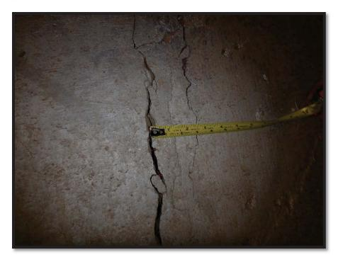
Photo 20 East Wall at 55-ft from south, showing 2-migrating cracks varying 1/8 to 1/2-inch and spalling
