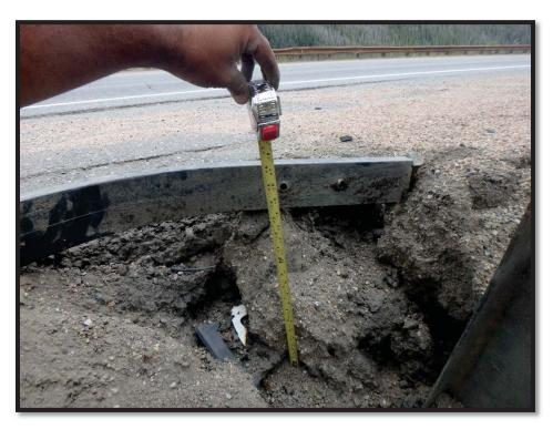
Photo 1 WB shoulder at guardrail, erosion 15-inches deep
