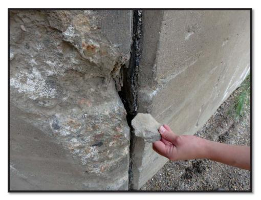
Photo 5 NW Wingwall at culvert joint, significant spalling
