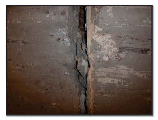
Photo 13 West wall at 44-ft from north, spalled and exposed rebar
