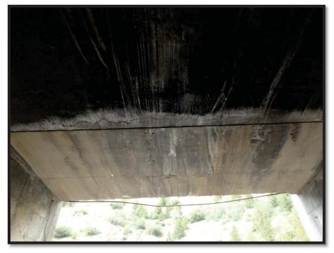
Photo 10 North End showing delamination/efflorescence and scrapes from live load
