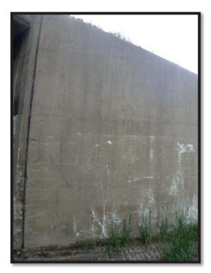
Photo 4 NW Wingwall showing diagonal 1/8-inch crack extending from joint to bottom
