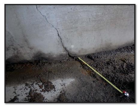
Photo 23 East Wall at 22-ft from south, showing diagonal shear crack ranging from 1/8 to 4-inches, migrating from wall into bottom slab
