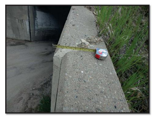
Photo 3 NW Wingwall showing sealed fracture, 4-iches of displacement
