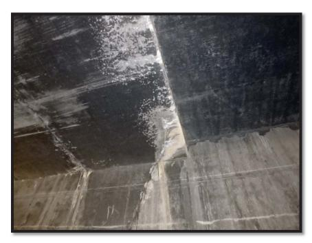
Photo 16 Top Slab at 85-ft from North (WB median) showing 1/2-inch to 2-inch shear crack migration from top slab down through wall
