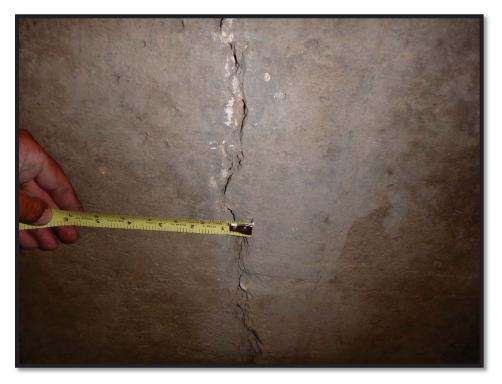
Photo 12 Close up of 1/4-inch crack from Photo 11
